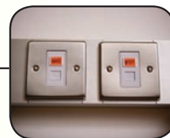
Face plate Label socket outlets, network points and telephone extension faceplates for quick identification.
